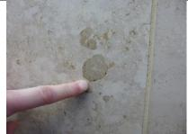
A black Spanish limestone, Nero Marquina, is Mid-Cretaceous in age and comes from Marquina, in the Basque country of NE Spain. It is a bituminous limestone with a micritic matrix. This rock has been weakly deformed, evidenced by the excellent conjugate sets of *en echelon* tension gashes, infilled with white calcite
